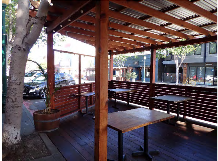
Parklet roof structure
