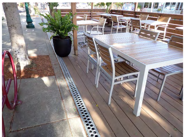
Parklet threshold flush to sidewalk
