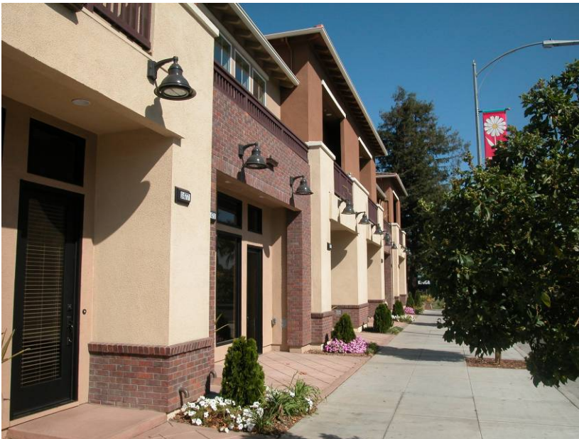
Example of live-work building
