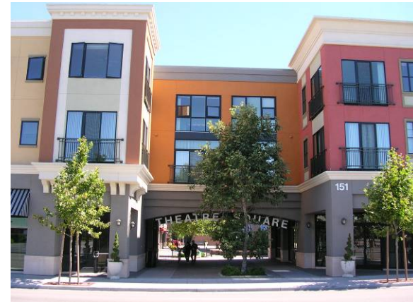
Example of a cut-through that is covered by the second floor of the building.
