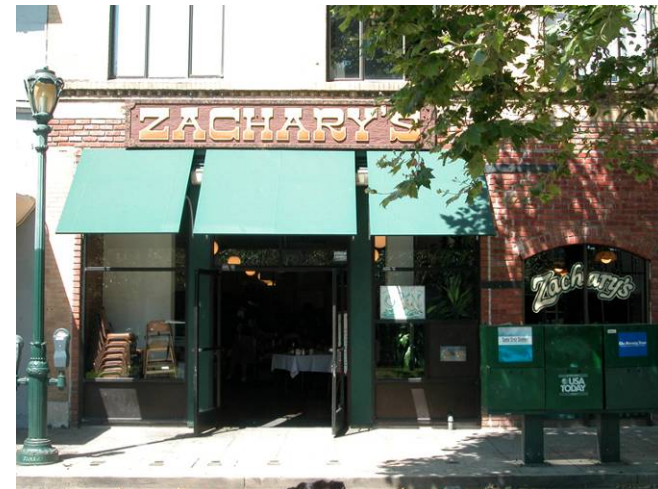
Example of a storefront sign
