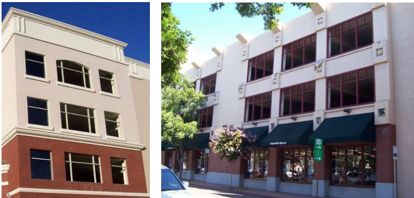
Examples of appropriately designed parking structure facades
