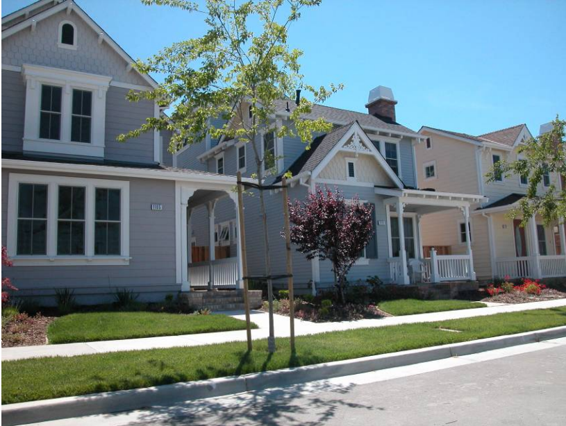
Examples of cottage house buildings
