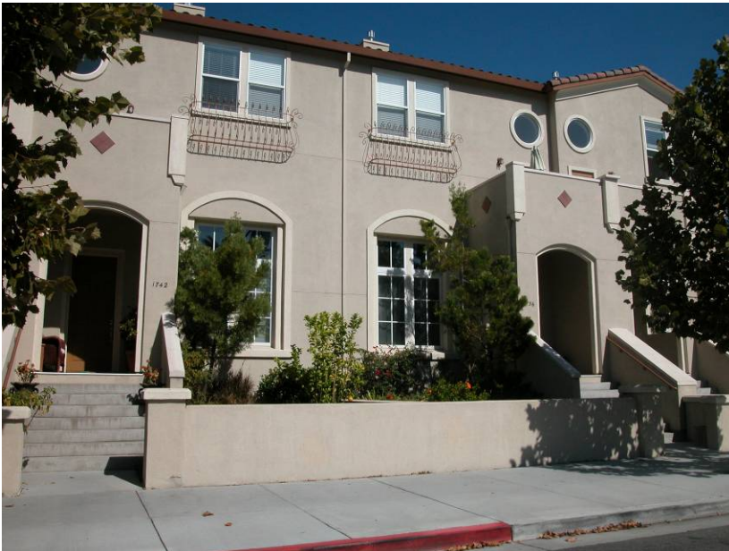
Examples of in-line townhouse buildings
