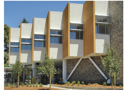
+ Horizontal sun shade with light shelf at south-facing windows.
