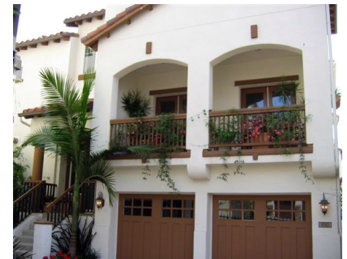
+ Balcony railings match the building architectural style.
