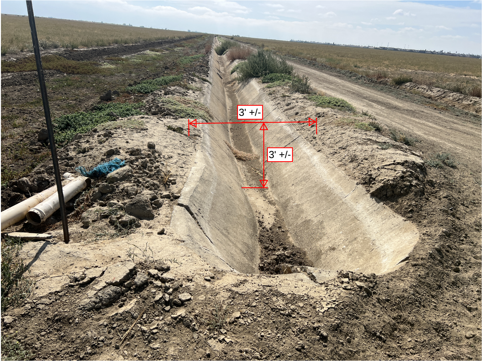
FIGURE 1 - EXISTING CONCRETE LINED IRRIGATION CHANNEL
